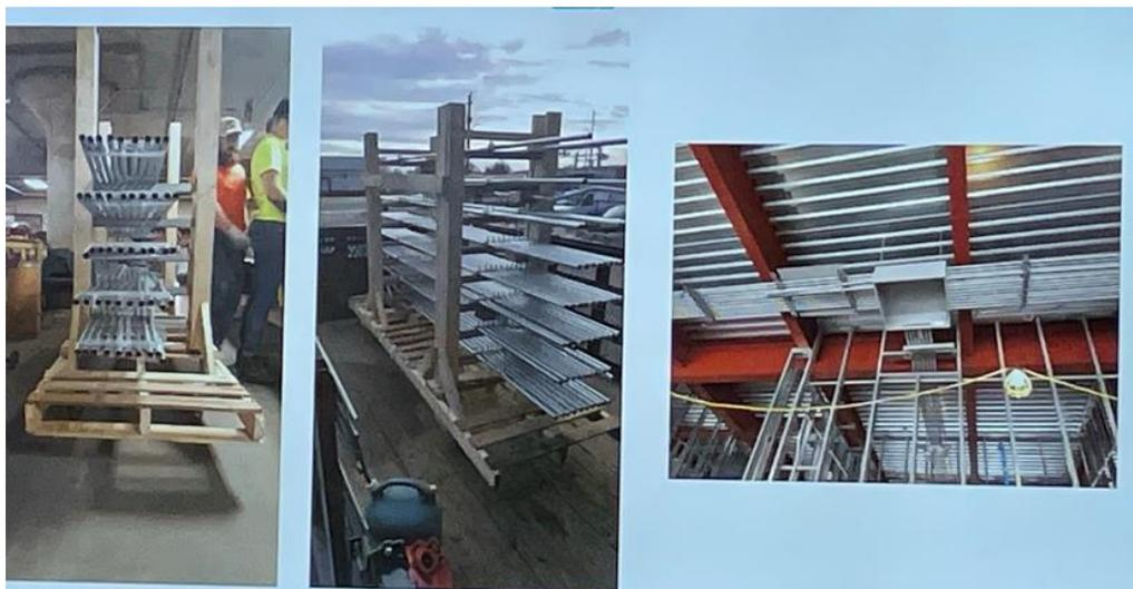
requirements, was commonly used to improve field installation rates. The racks were typically set at 10-foot lengths with two support struts, spaced five feet apart, as a size found to be manageable for a two-person crew. On one example project visited, the foreman cited installing an entire run of 10' racks across 120 feet of space within one day of work by a two-person crew. The project was a retail store with approximately 20' roof height.
